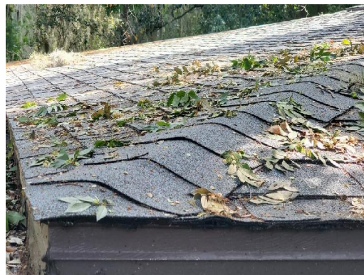
923-1 Asphalt Shingle/Tar Typical Exterior Roof
