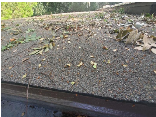
923-2 Rolled Roofing Carport/Enclosed Porch
